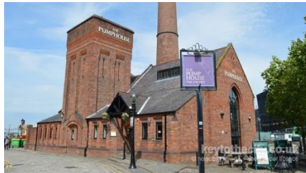
The Pump House
